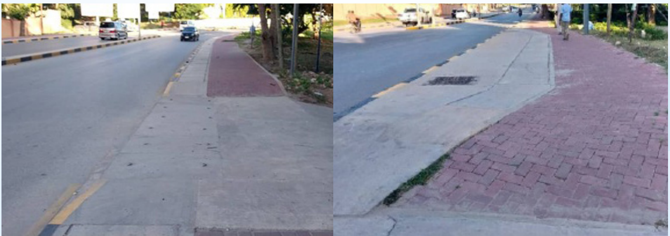
Pictures of Airport – Mnazi Mmoja road, designed with pedestrian walkways where people with disabilities use conveniently.
