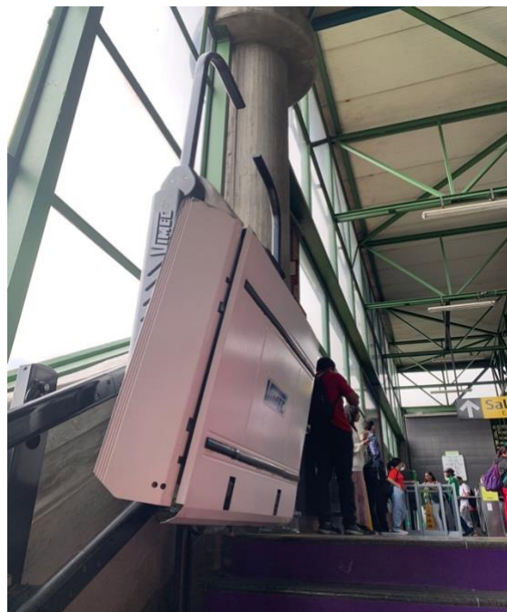
Platform lift at stairs at Metro Station
